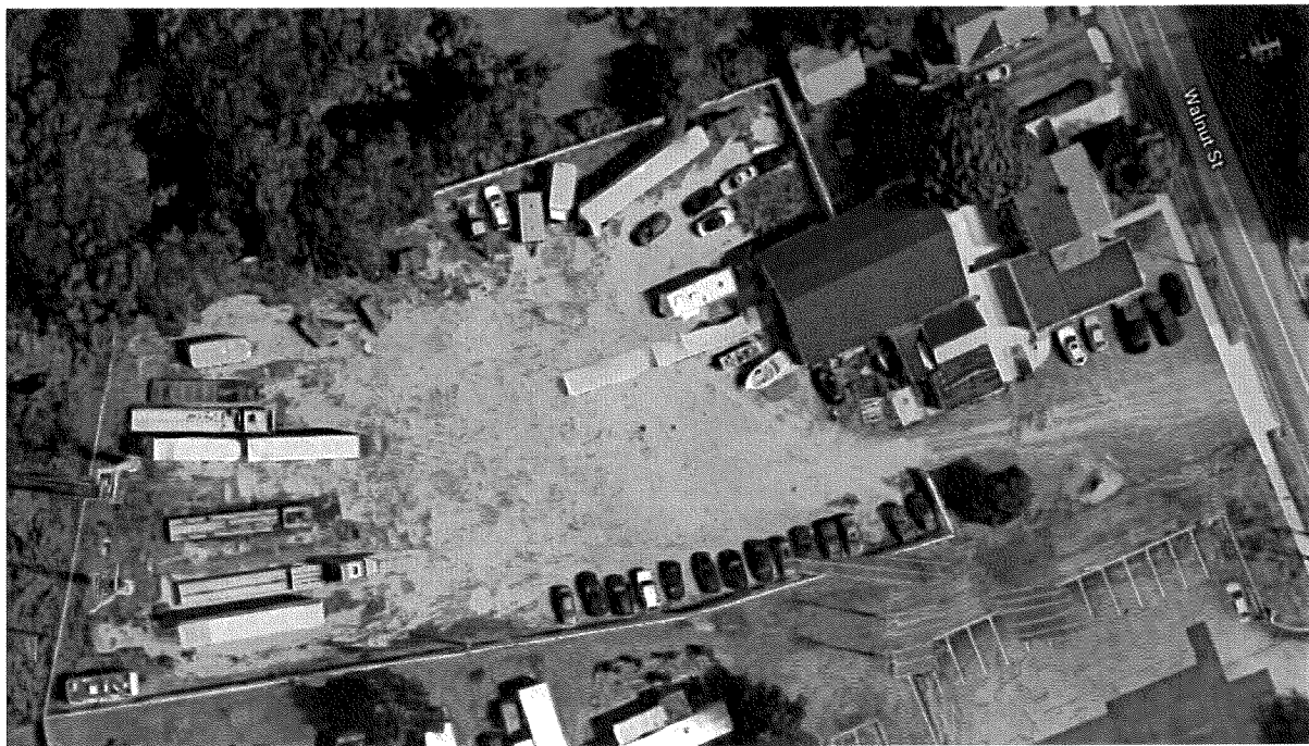
Aerial photo of project site, Imagery @2019 Google – hard pack gravel used for parking by BBB Automotive Inc.
