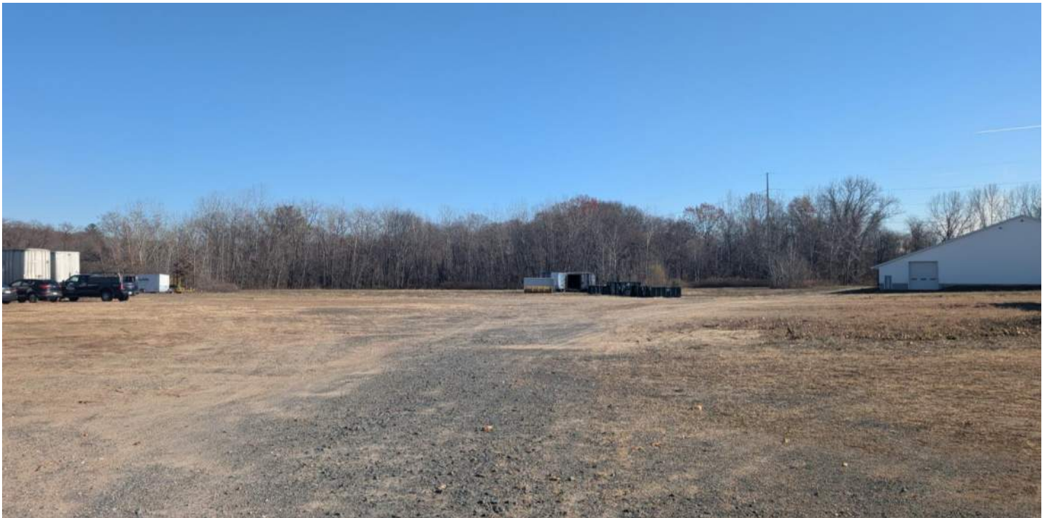
Photo 6: View of proposed substation area in the southeast corner of the site. Facing southeast. Surveyed 11/19/2025.
