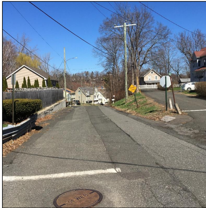
Photo No. 1. Project begin location at the intersection of Moore Street and High Street. The current roadway width of Moore Street varies from 16 ft to 25-ft and will be improved with a uniform 18 ft width and increased pervious area.
