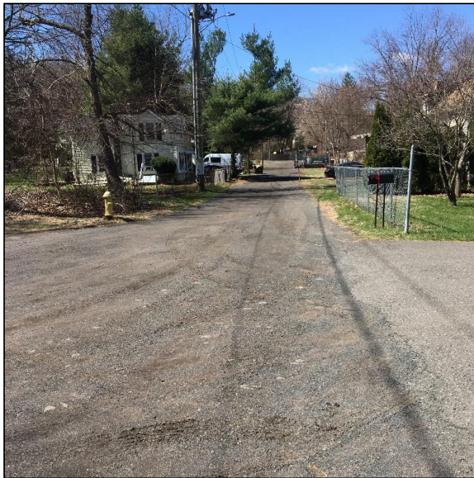
Photo No. 10. Westward view from the east end of Valley Street (east). The proposed roadway surface improvements will include an asphalt paved surface at the same surface elevations.
