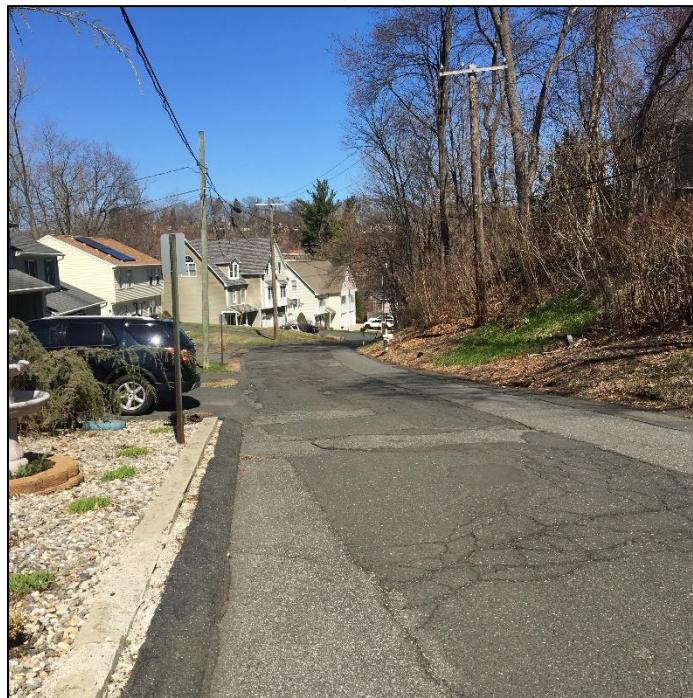
Photo No. 2. Typical view of deteriorated pavement near 54-56 Moore Street. Location is outside of environmental resource areas or buffers.
