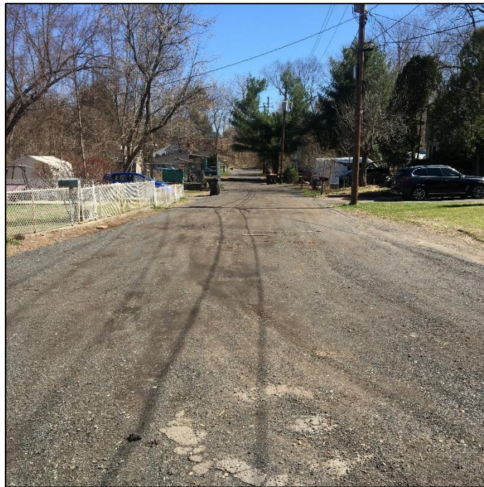
Photo No. 4. View of Valley Street (east) from the intersection of Moore Street. Note the 33-ft wide gravel road width near intersection. The majority of Valley Street (east) is within the 200-ft Riverfront Area.
