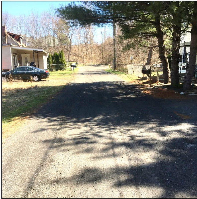
Photo No. 7. View of Valley Street (east) gravel road surface. A 125-ft long segment of FEMA Zone AE Floodway is mapped in the area and to the north (left of photograph).
