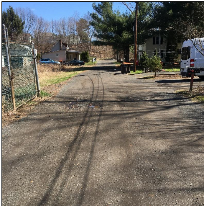
Photo No. 6. View of Valley Street (east) gravel surface and location of sanitary sewer pump station (to left chain link fence).
