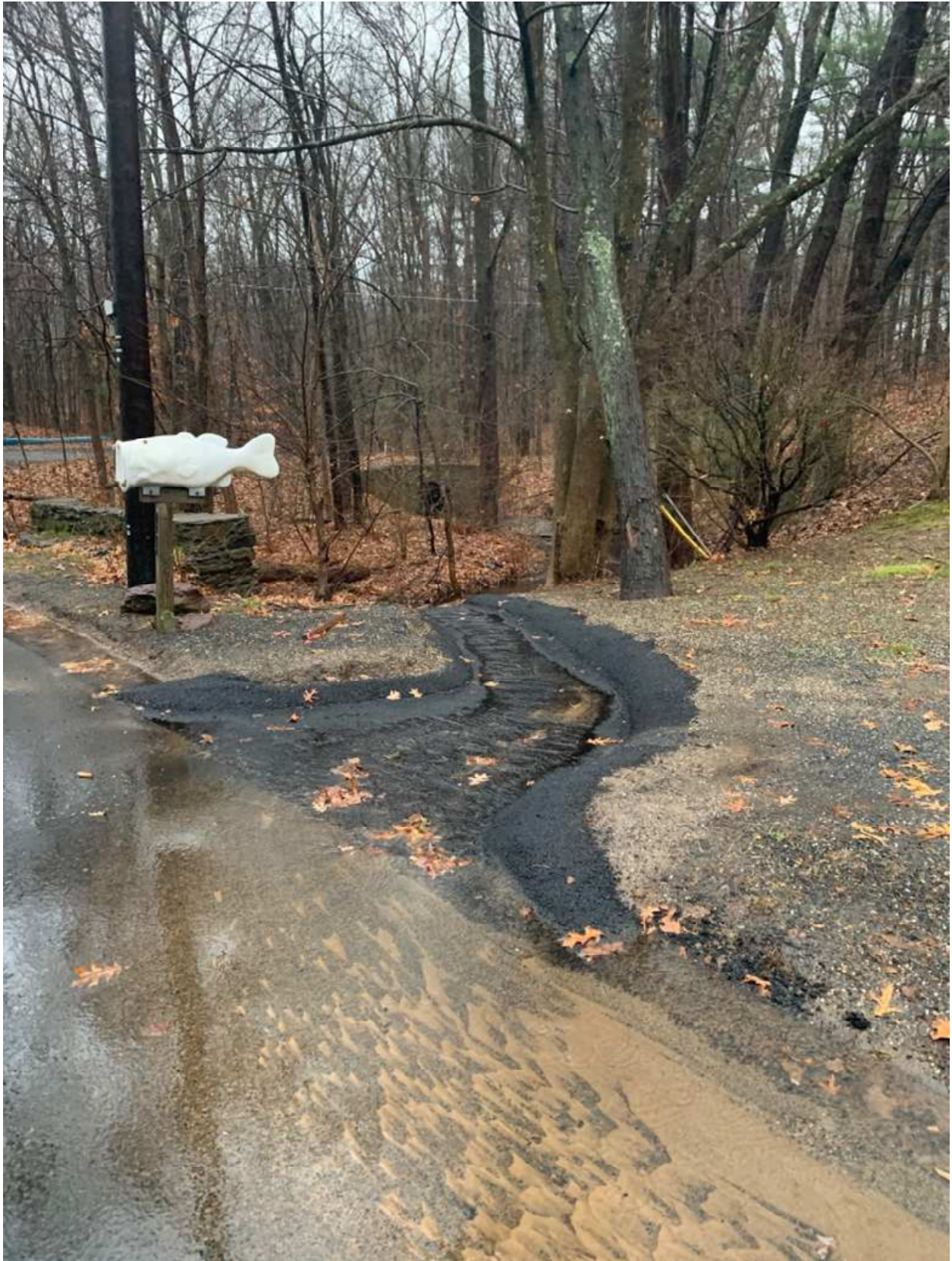
South West Street stream crossing with paved swale – December 1, 2020
