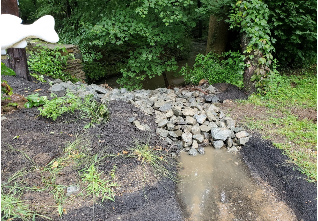
South West Street stream crossing, Riprap installed by DPW to reduce erosion – August 19, 2021
