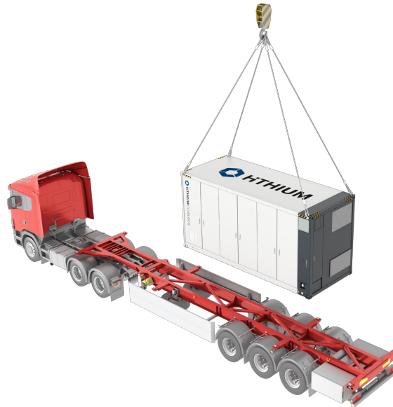
Fig 4-3 Hoist the ESS Container to the Transport Vehicle
