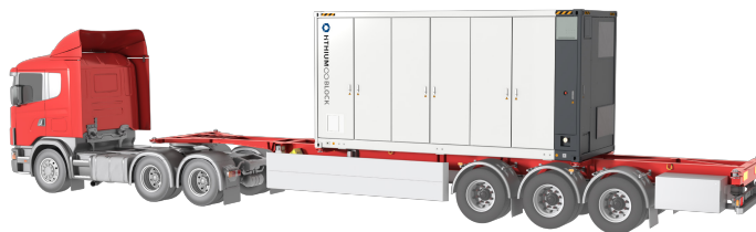
Fig 4-4 Place ESS Container to the Target Position
