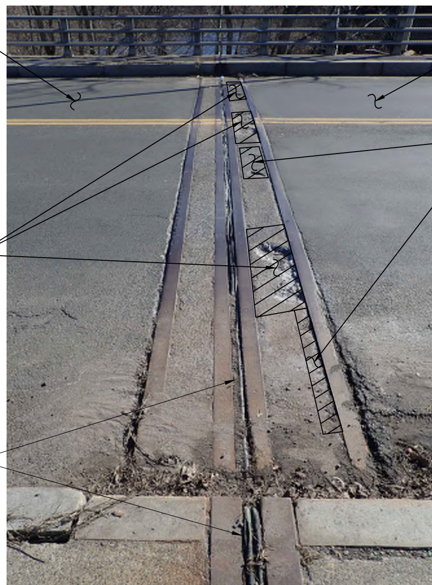
NORTH ABUTMENT BRIDGE JOINT LOOKING EAST
