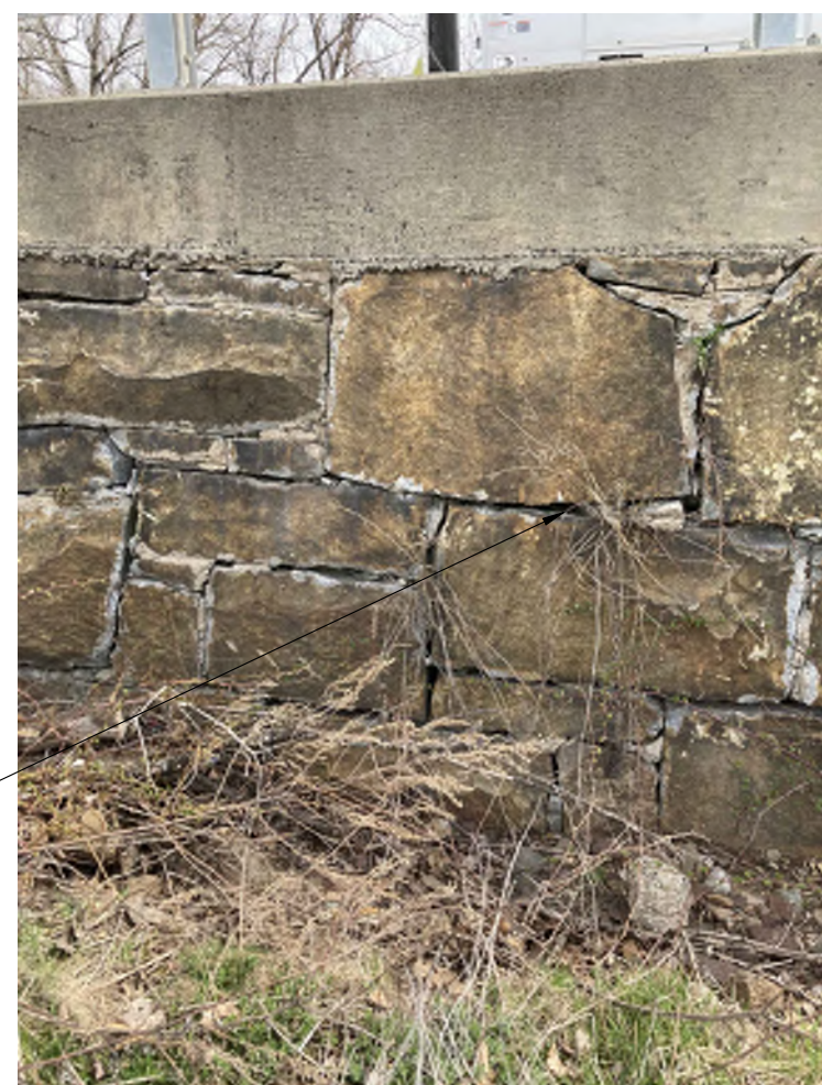
MASONRY WALL REPAIR
