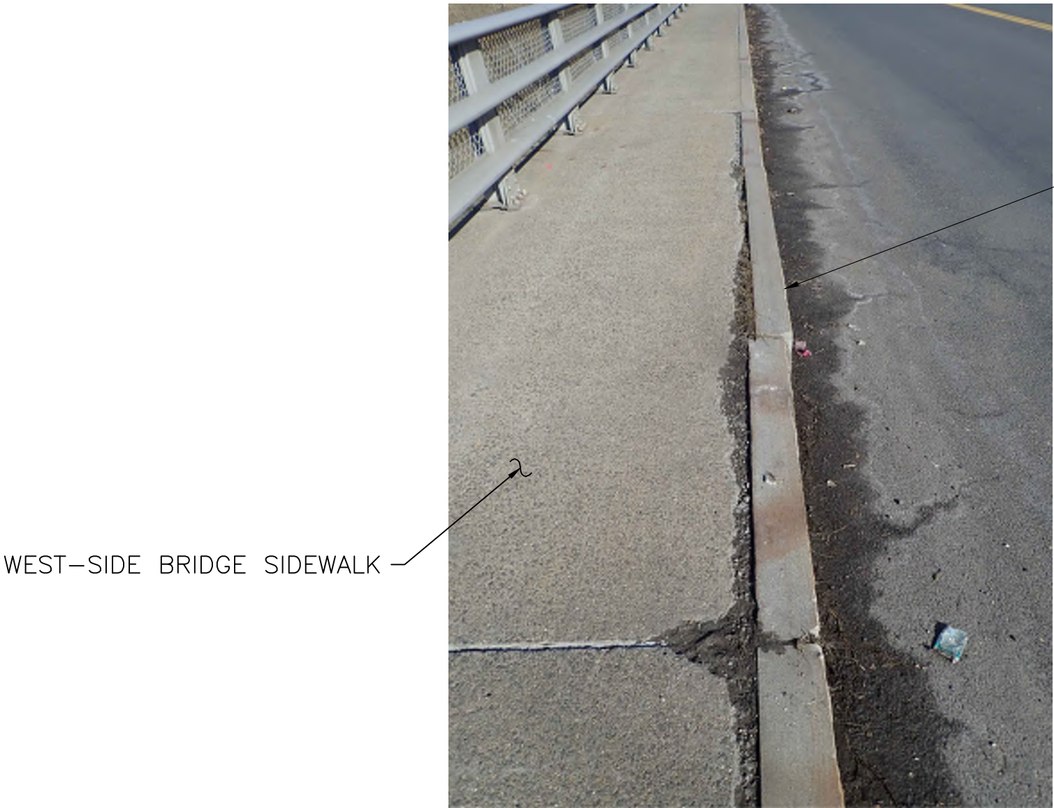
BRIDGE GRANITE CURB RESET
