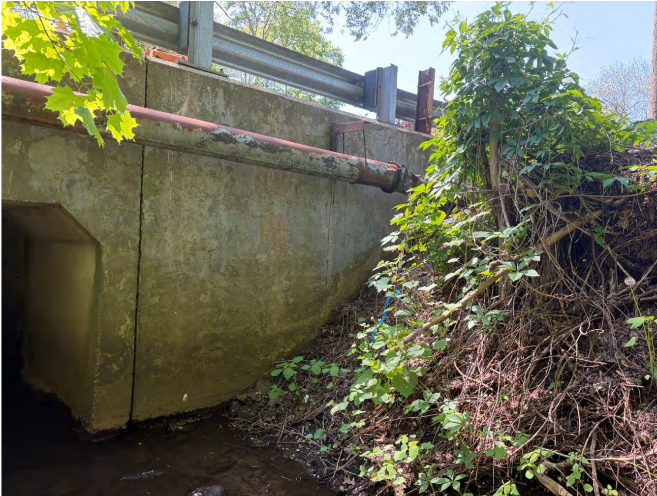
Photo 9. Southerly view of steep western slope on north side of Adams Street.
