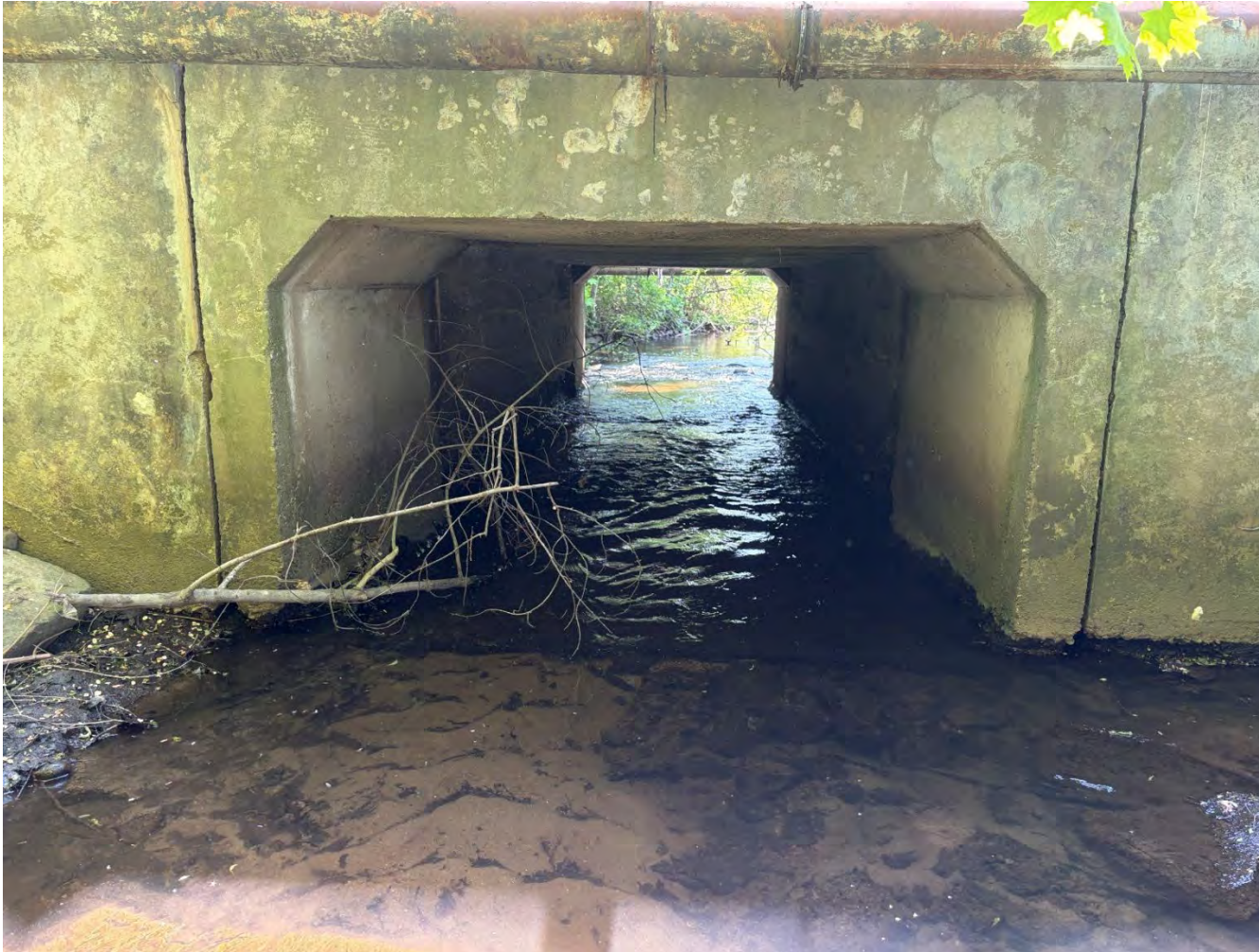
Photo 8. Southerly view of culvert on north side of Adams Street.
