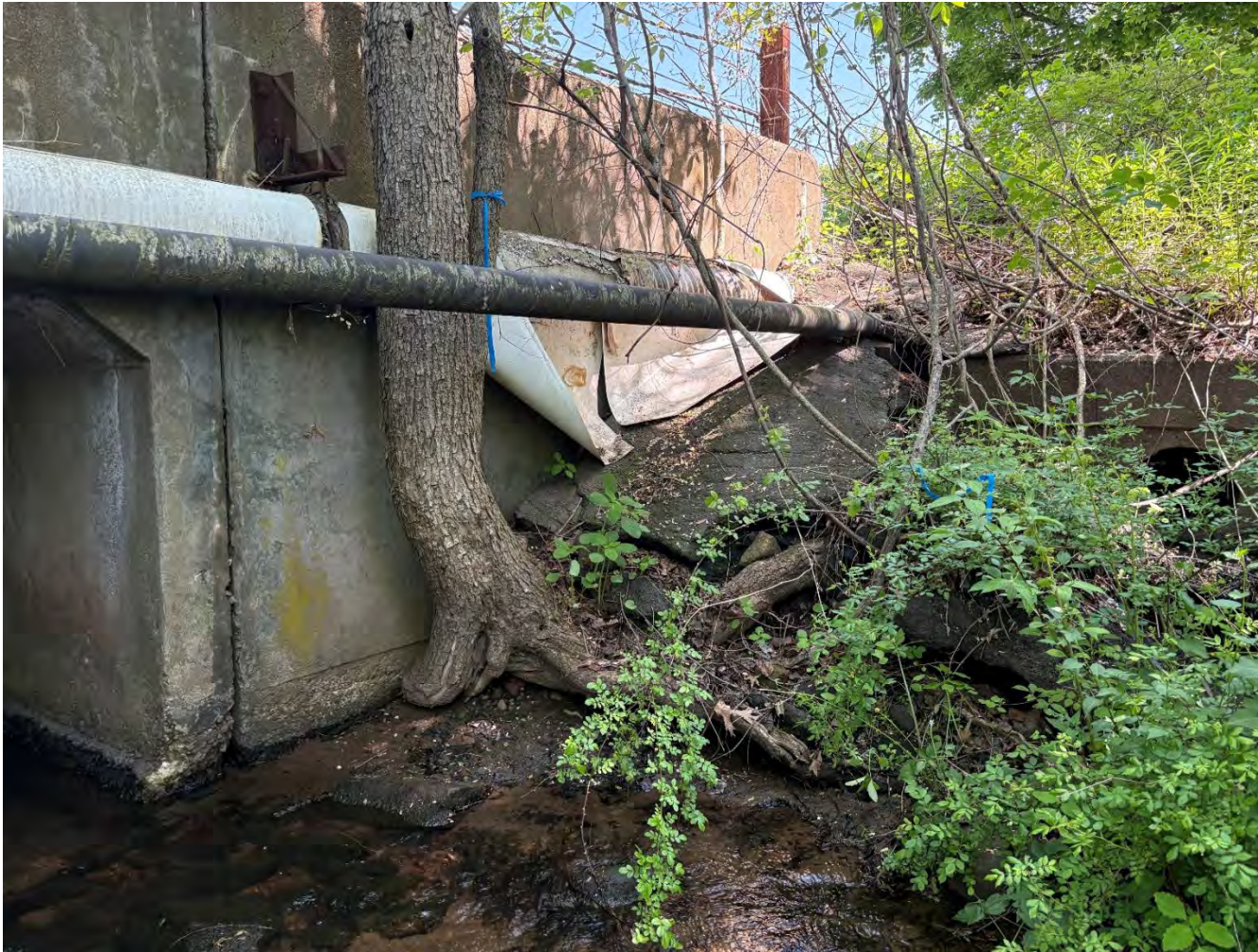
Photo 4. Easterly view of existing drainage outfall and paved stormwater conveyance on slope abutting culvert headwall. View of existing utilities crossing the culvert.
