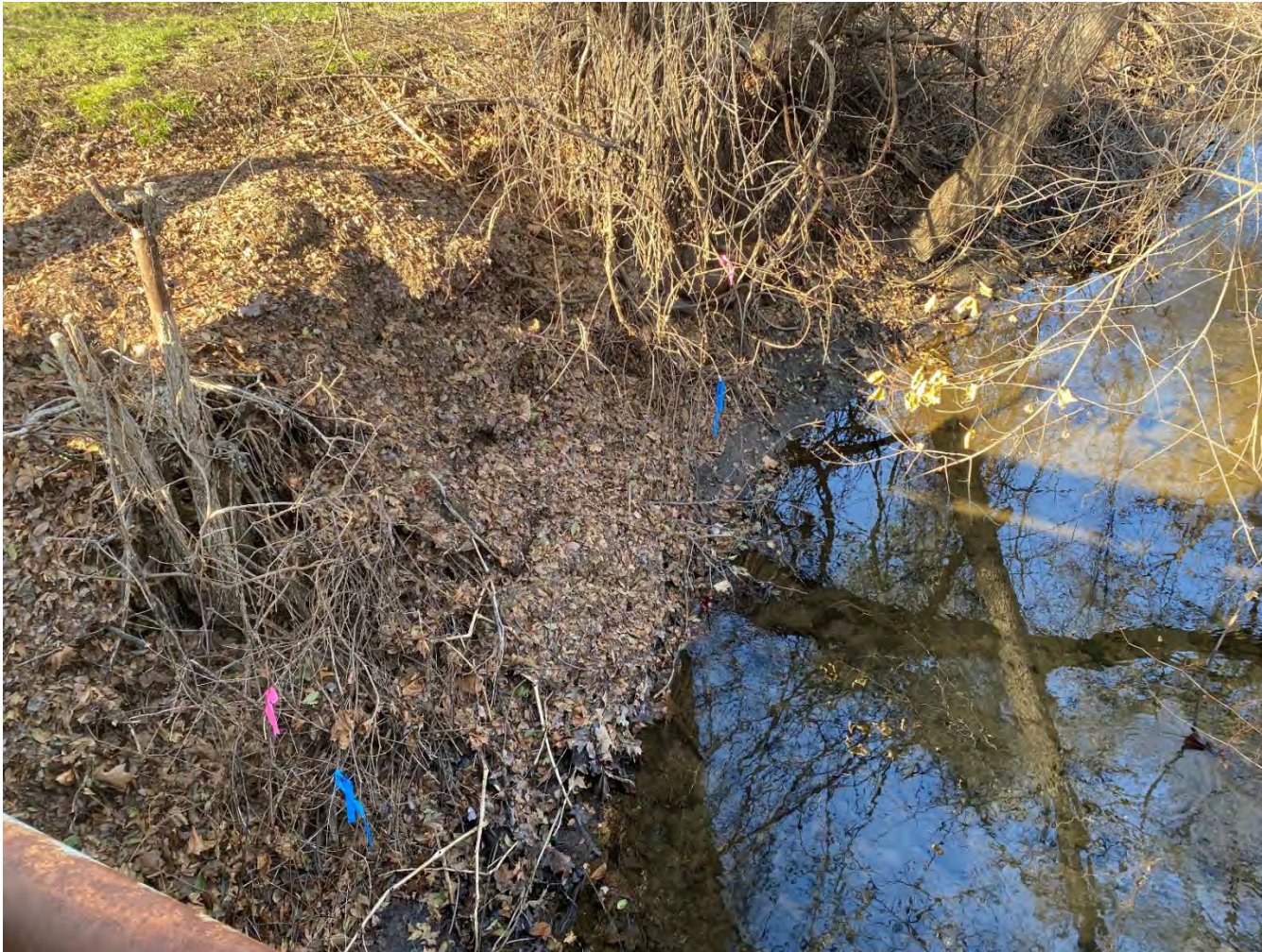
Photo 10. Northerly view of steep western slope on north side of Adams Street.
