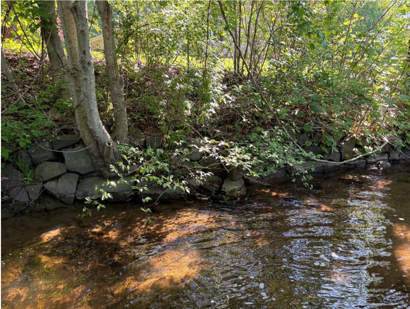
Photo 6. View of eastern Bank with placed rip rap on lower slope.
