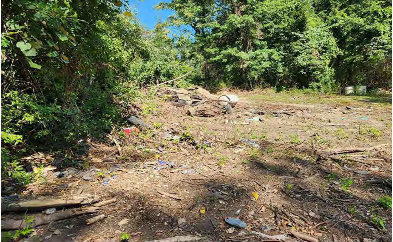
Photo 11. Trash and debris strewn across the western edge of the site.
