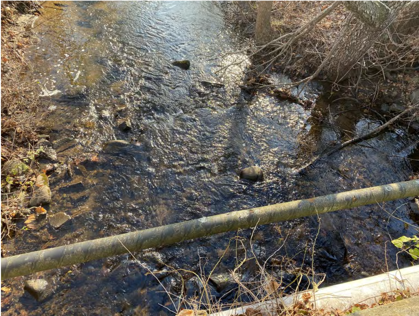
Photo 7. View of cobble, rocks, and small boulders at outfall of culvert. Streambed transitions to sand and fine to coarse gravel.
