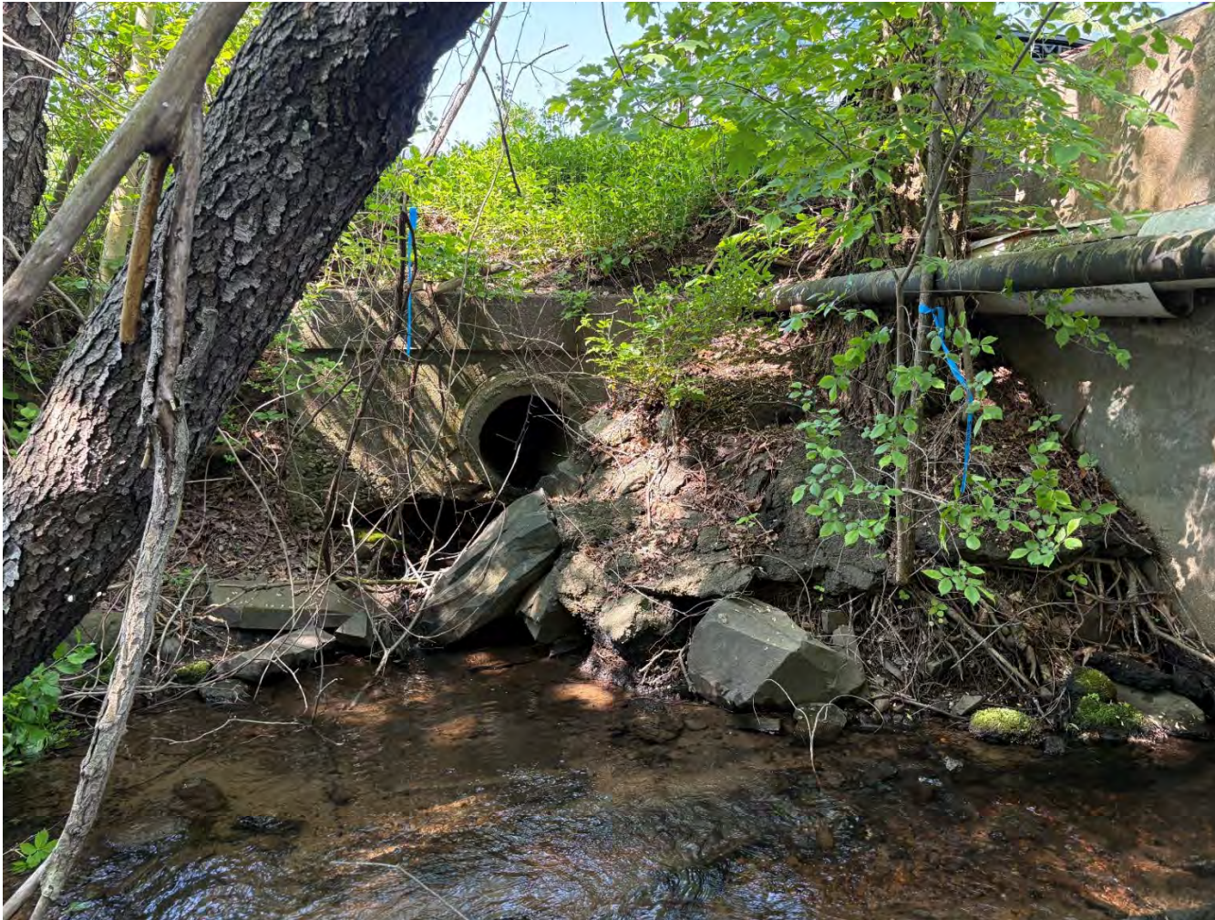
Photo 3. Westerly view of existing drainage outfall with placed rip-rap and paved stormwater conveyance on slope abutting culvert headwall.
