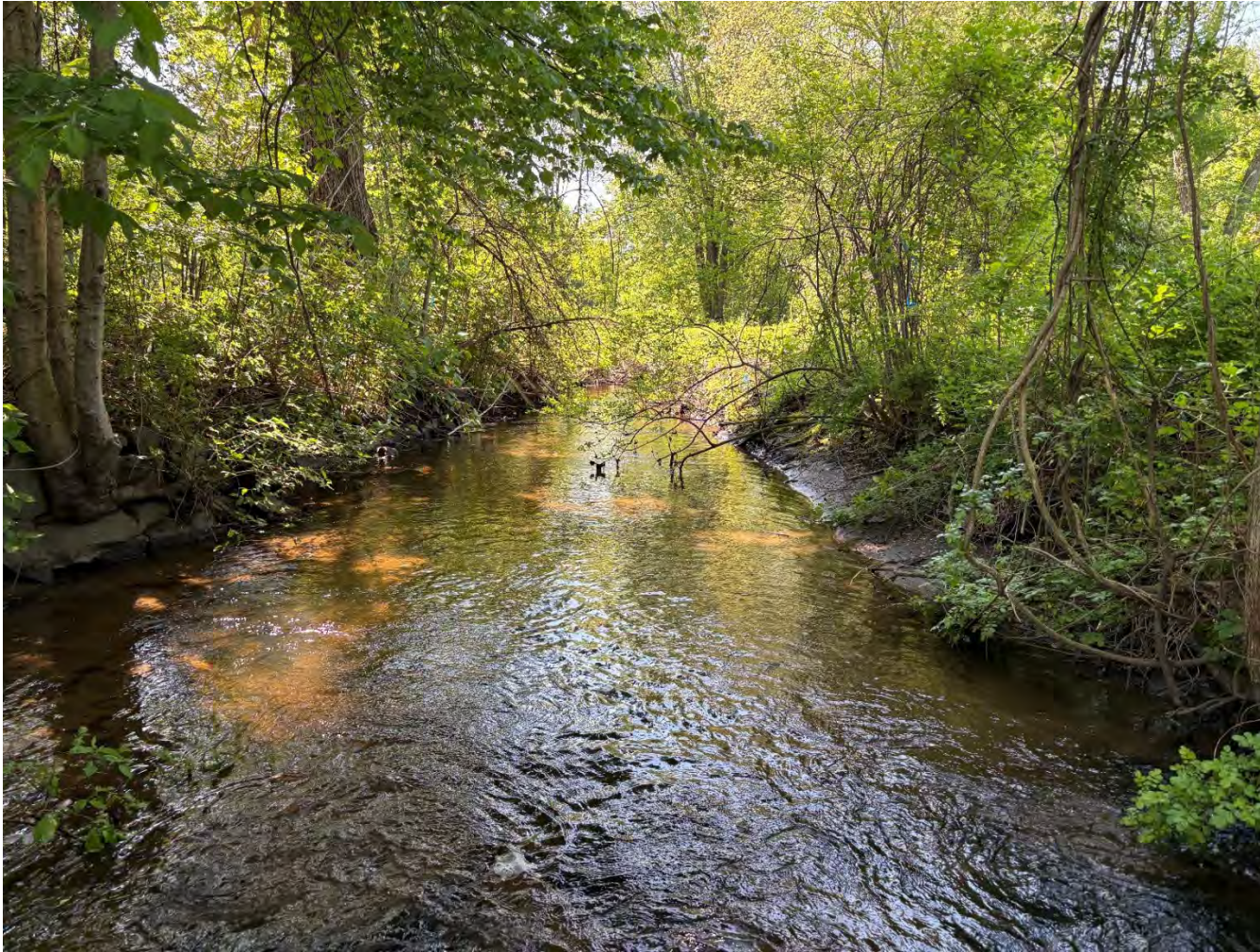
Photo 5. Southerly view of Three Mile Brook immediately downstream of culvert. Placed rip rap on lower east Bank (left).
