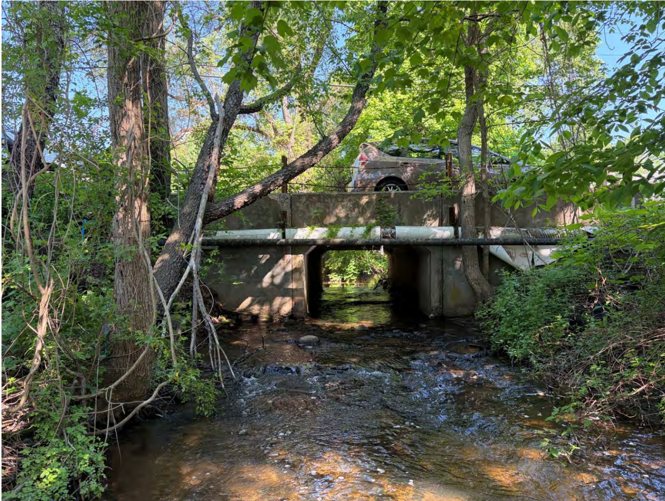
Photo 2. Northerly view of Three Mile Brook and culvert on south side of Adams Street.
