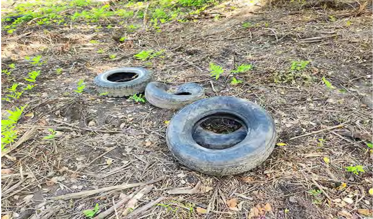
Photo 5. A few of the many tires observed on the site within the cut or cleared area.
