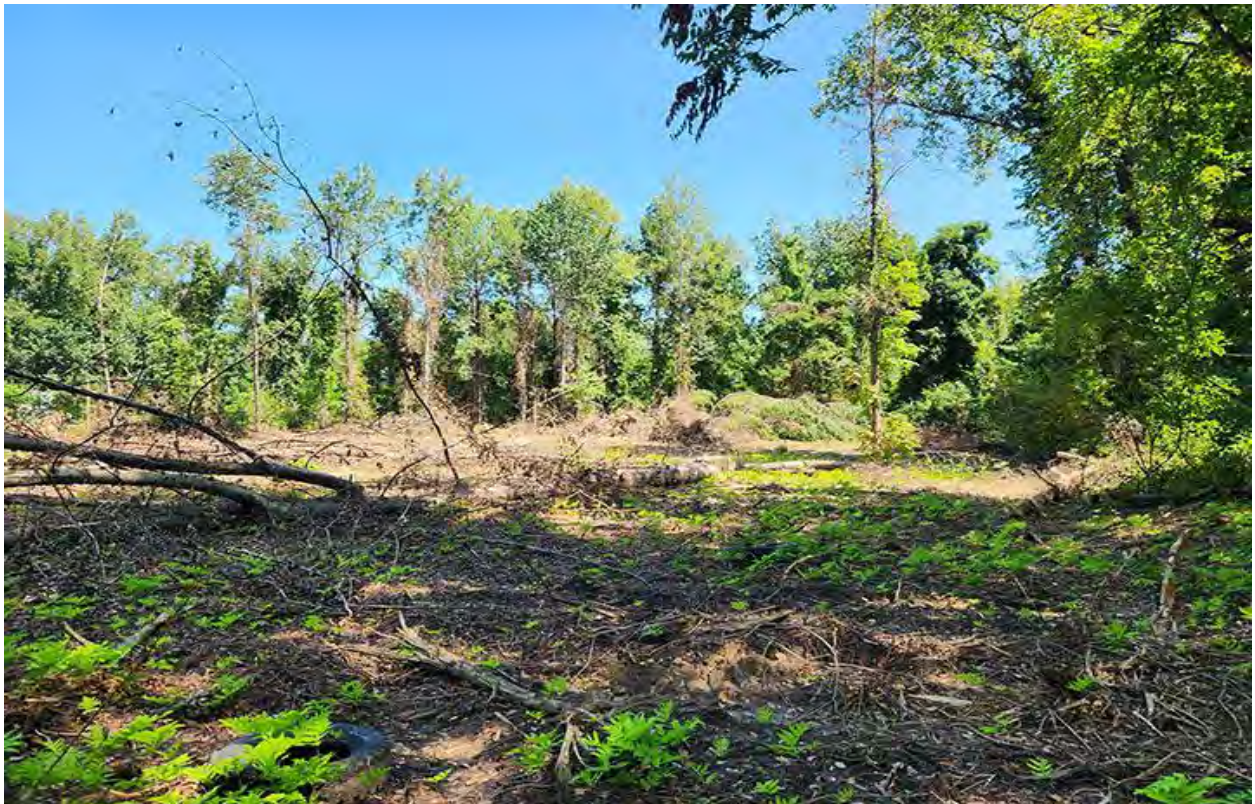
Photo 4. Cleared area of Wetland A and floodplain to the upper left of photograph.
