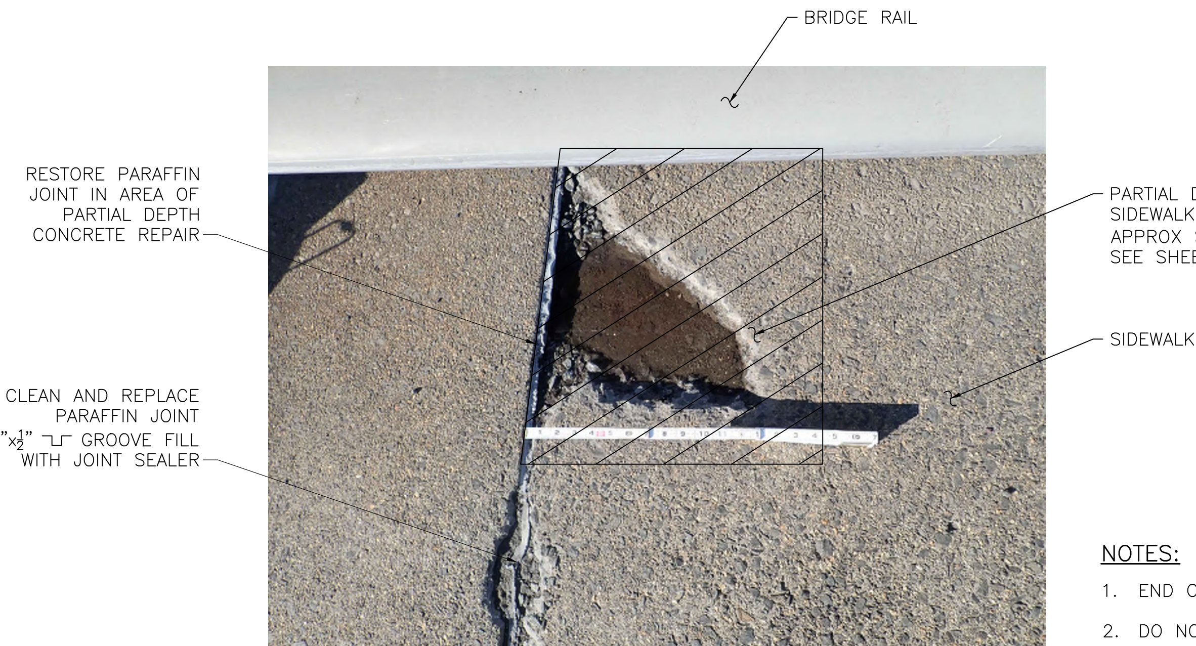
PARTIAL DEPTH CONCRETE SIDEWALK REPAIR
