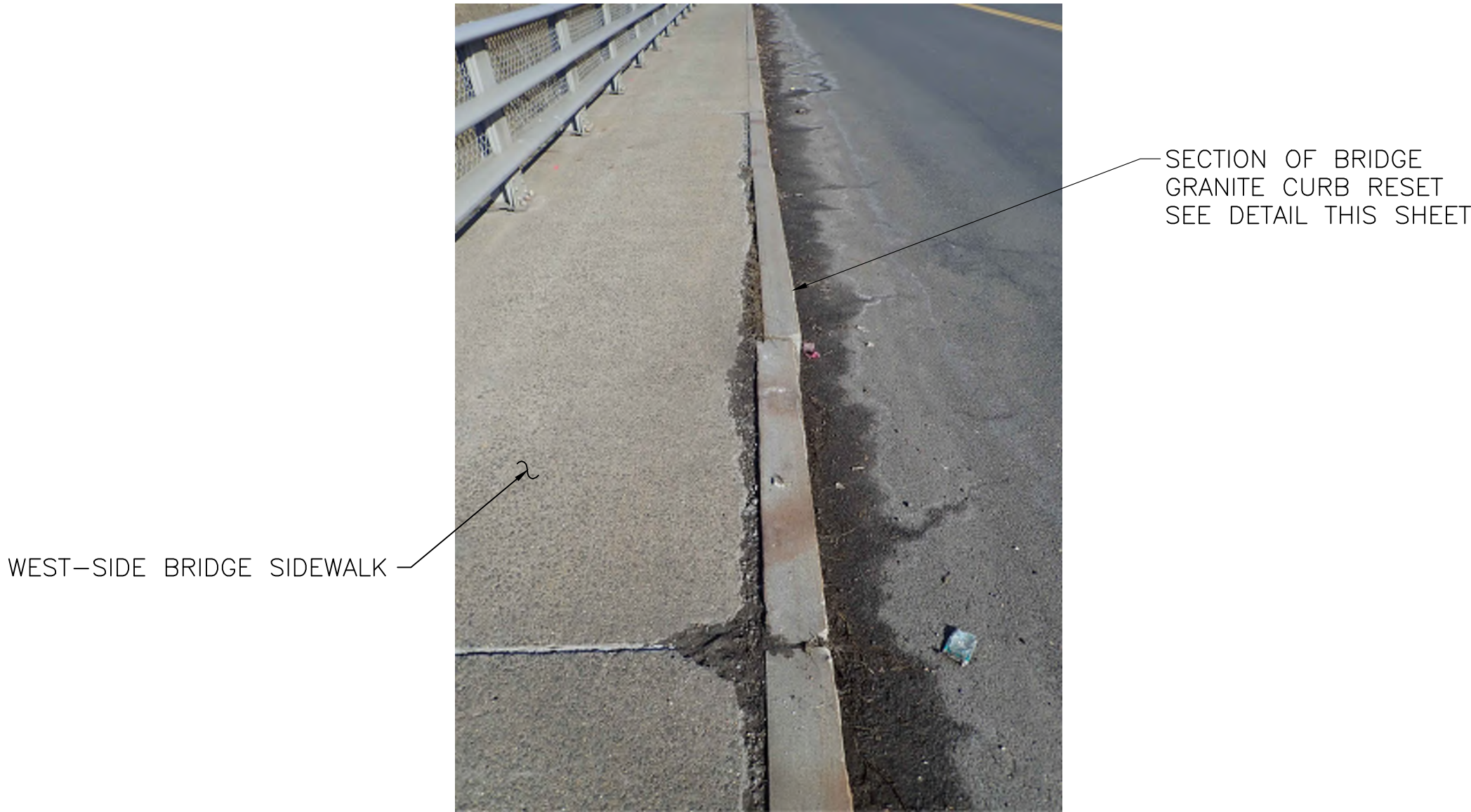
BRIDGE GRANITE CURB RESET
