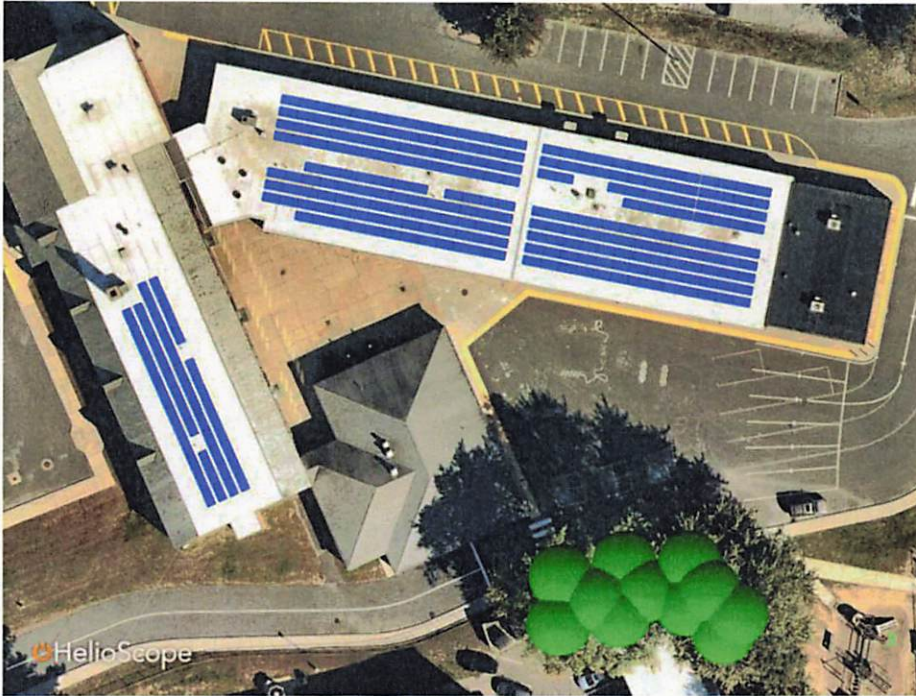
Granger Elementary School
