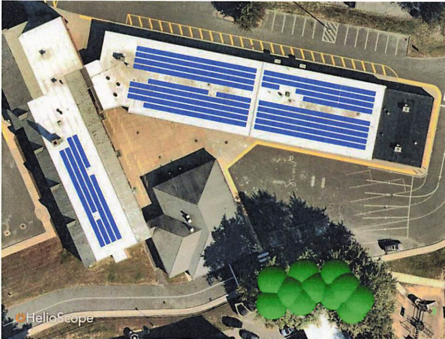
Granger Elementary School
