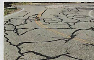
crack sealing
