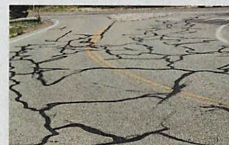
crack sealing
