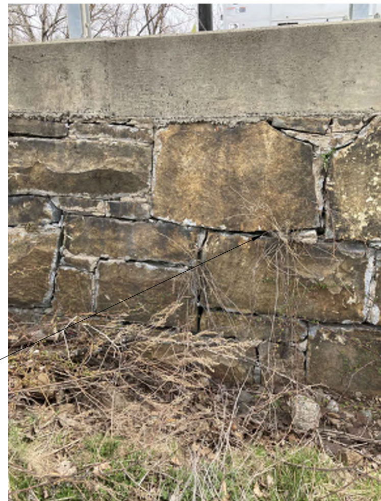
MASONRY WALL REPAIR
