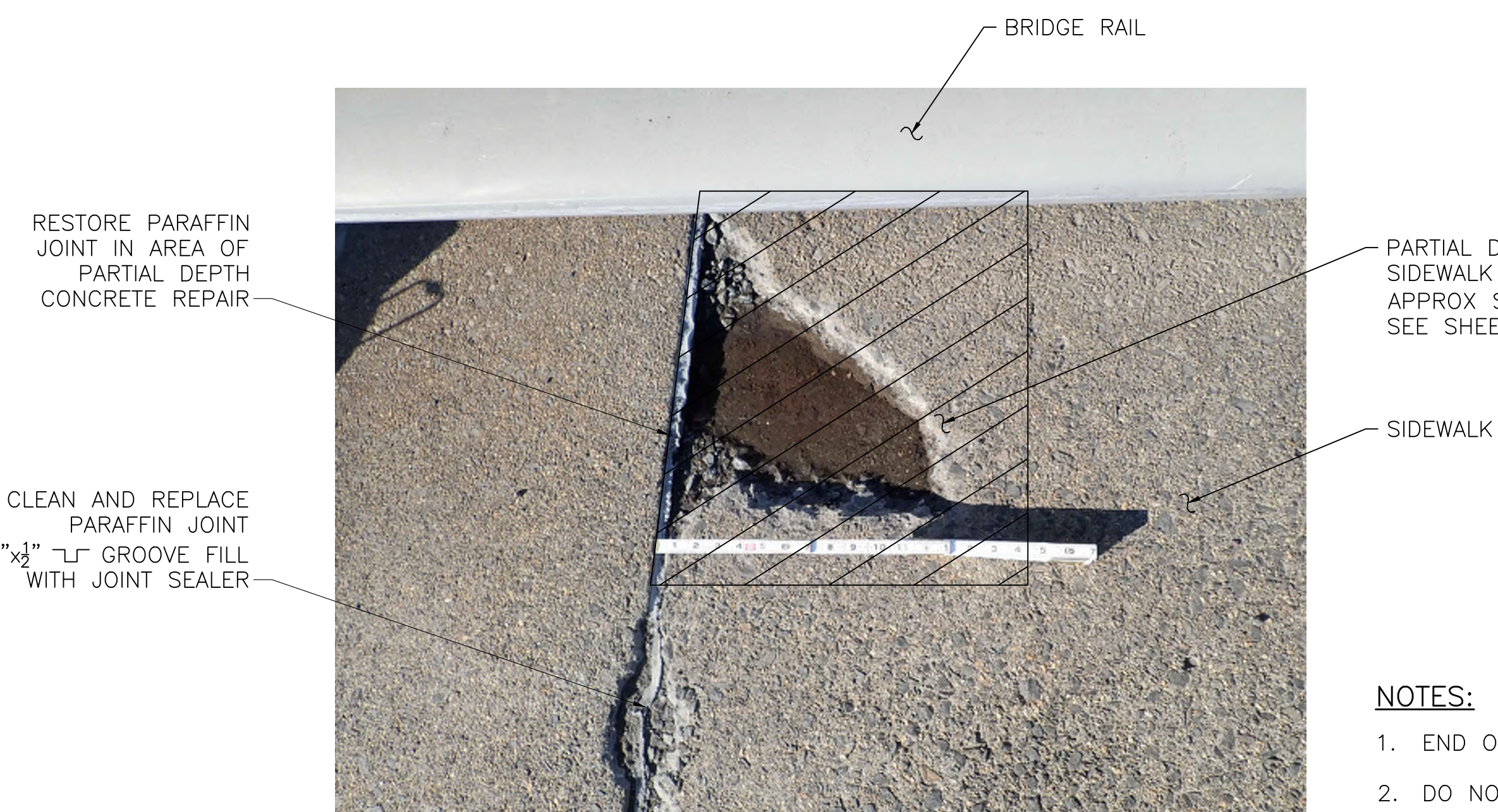
PARTIAL DEPTH CONCRETE SIDEWALK REPAIR
